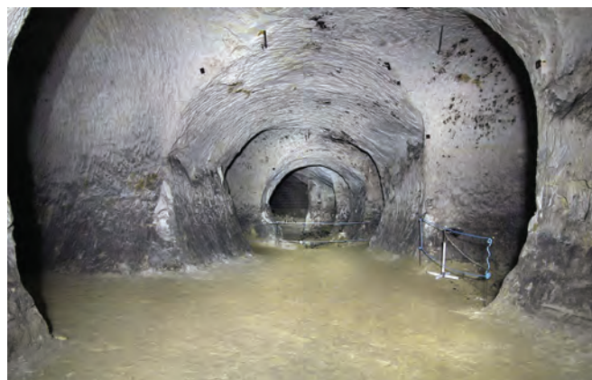
Tunnel Road West. Photo Nick Catford
